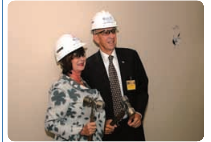
Pam and Les Muma are all smiles after taking a sledgehammer to the wall, symbolizing the beginning of construction of the Jennifer Leigh Muma Neonatal Intensive Care Unit.
